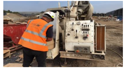
(9) Fibre are added to truck by blowers while mixing at full revs
