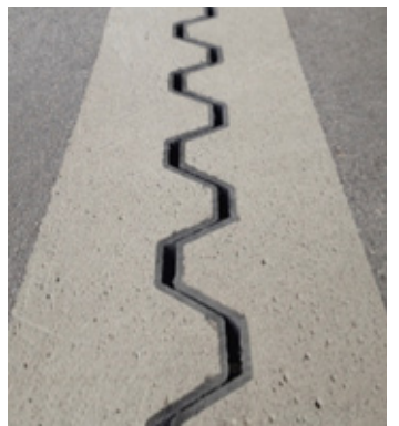
Concrete slab after repair
