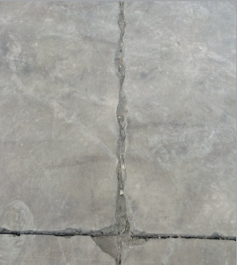
Damaged concrete slab before repair
