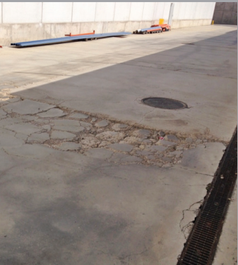
Damaged concrete slab before repair
