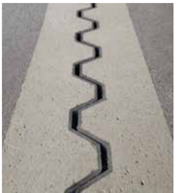
Concrete slab after repair
