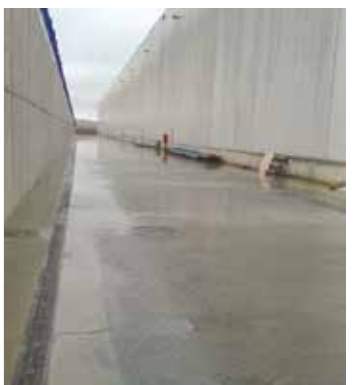
Concrete slab after repair
